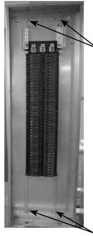
Figure 3. Removing interior hardware
