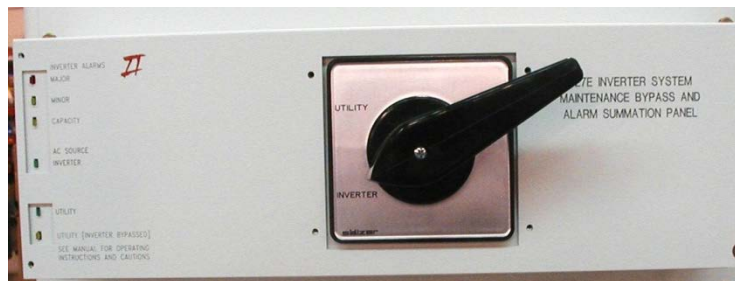
FIGURE 2-2: Front View of the 6310408P-1 30KVA Bypass Panel
