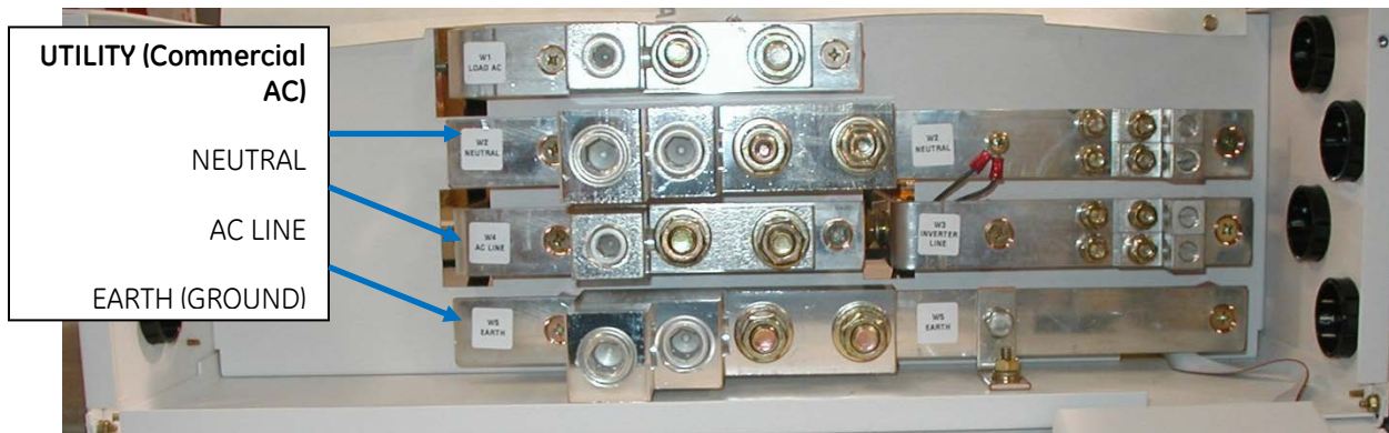
Figure 3-3: Commercial AC Input Connections (view from top)
