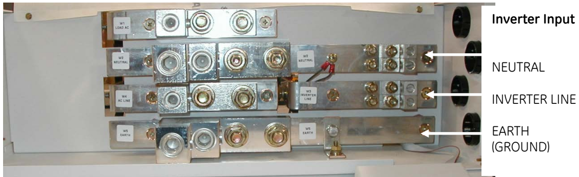
Figure 3-4: Inverter Input Connections
