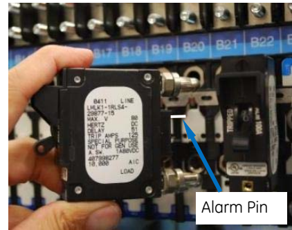
Correct Breaker orientation for insertion
