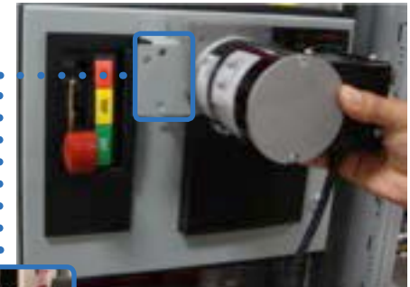
Above: Racking motor mounted to AFM unit
