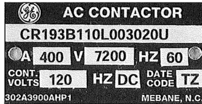
Figure 1. High-Voltage Contactor Nameplate
