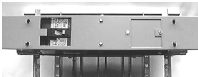
Figure 5. Breaker cover installed on the filler supports for SE, SF, TFJ, TFK, THFK, and TFL breakers.
