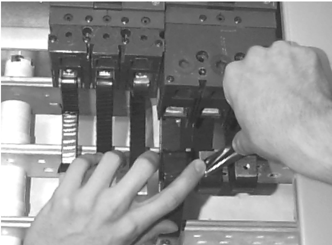
Figure 8. Applying insulating tape to unused strap contact surfaces.
