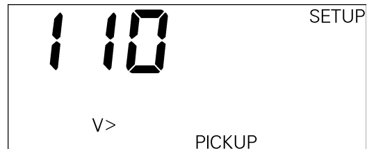
Figure 31. Trip Unit display for overvoltage relay pickup.
