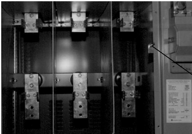
This interlock prevents inadvertent closure of switch if the enclosure door is open. When the door is closed, the push rod is depressed by the door to move the safety latch out of the blocking position. See Figure 14.
