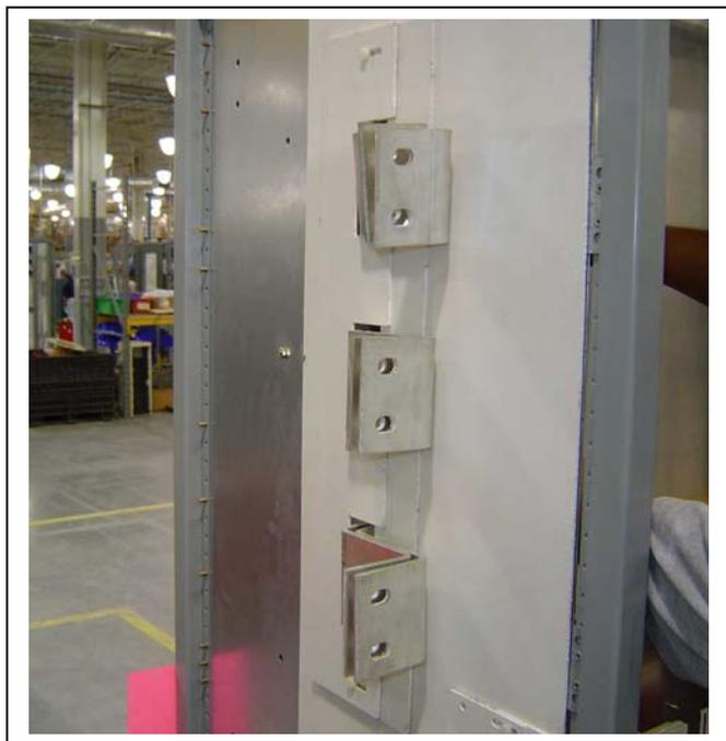
Second, attach the next section and make the bus bar holes align with the splice bar slots. There is a removable cut out for temporary removal during the splicing of the section.
