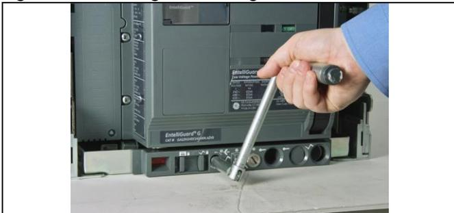
16. Continue rotating the racking handle clockwise until the position indicator first shows TEST, then CONNECTED. When approaching the CONNECTED position, effort to turn the racking handle will increase as the clusters engage with the cassette-mounted contacts. If a motor spring charge or under voltage to release is installed, these may operate when approaching the TEST position.
