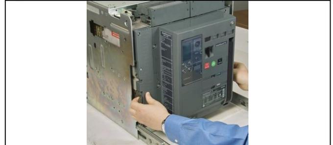
9. Push back both the extended rails of the cassette to the stowed position.
