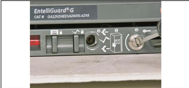
14. Insert the racking handle in the handle insertion hole on the cassette front panel.
