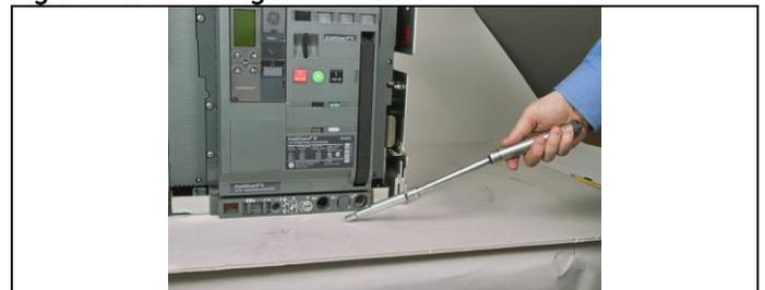
13. With a screwdriver, turn the racking handle shutter drive A clockwise (Fig. 3.14).
