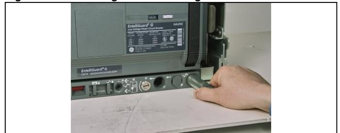
12. Pull out the torque bar from inside the handle and extend (Fig. 3.13).
