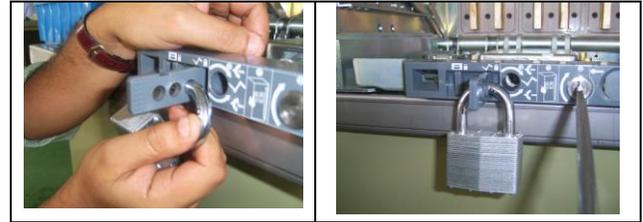
4. Using a screwdriver, turn the racking handle shutter drive A clockwise.
