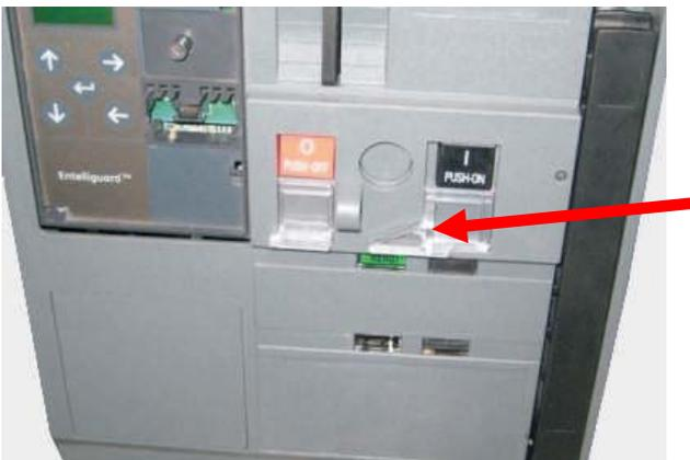
Figure 4: Fixing the screws
