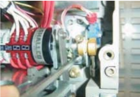
Figure 6. Assemble the Auxiliary switch
