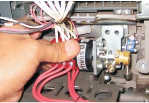
Figure 5. Remove the existing Auxiliary switch assembly
