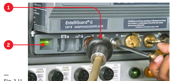
1. Racking handle 2. Breaker position indicator
