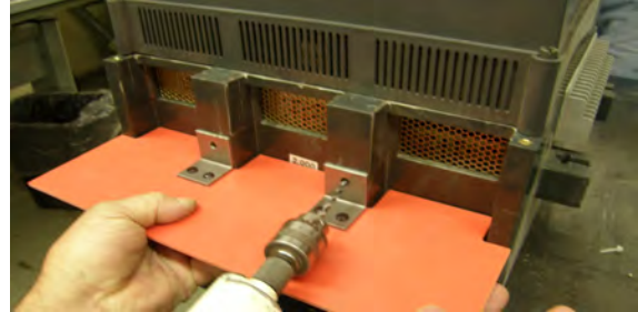
Figure 5: Mark the Area for Drilling Holes
