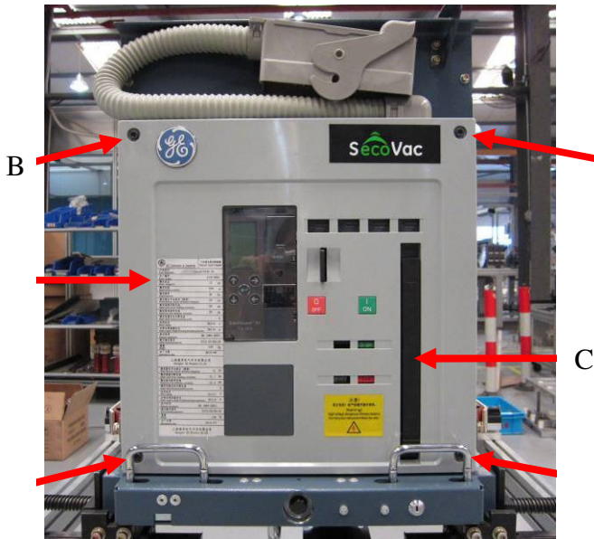
Figure 1. (A) Front Cover (B) Screw Removal (C) Handle Rotation
