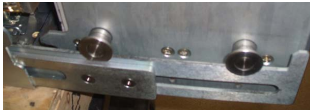
Figure 3.5. Circuit Breaker Rollers Straddled on the Loading Rails
