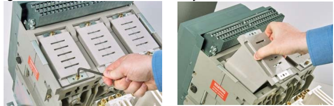
Figure 8.2. Arc Chamber Assembly Removal
