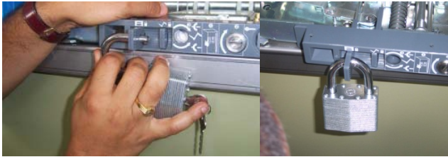
Figure 5.4. Padlock Insertion
