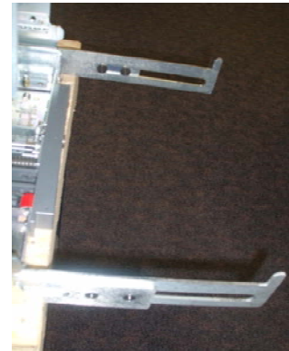
Figure 3.10. Cassette Rails Pulled Out for Circuit Breaker Unloading
