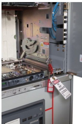
Figure 3.4. Racking Drive in the DISCONNECTED Position
