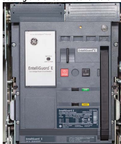
Figure 3.7. Setting the Circuit Breaker to OFF
