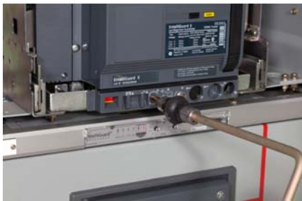
Figure 3.9. Turning the Racking Handle
