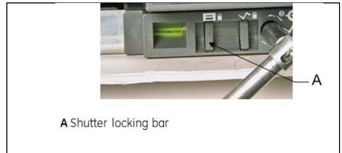
Figure 5.6. Shutter Padlocking
