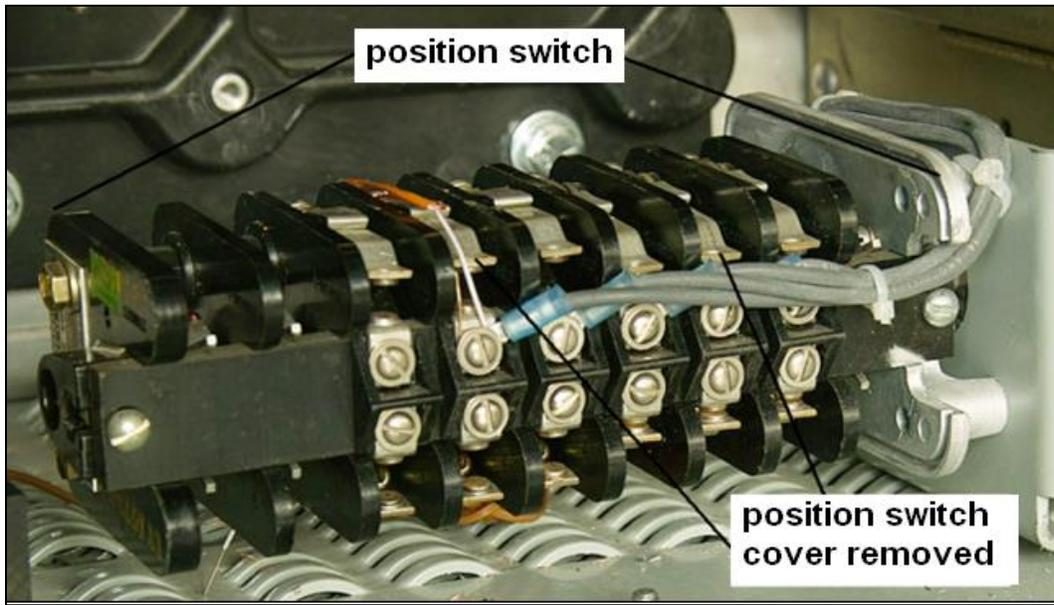
The mechanical subassembly comes with mounting hardware, lever, and bracket. Depending on the switchgear, this simple device is mounted in different locations.
