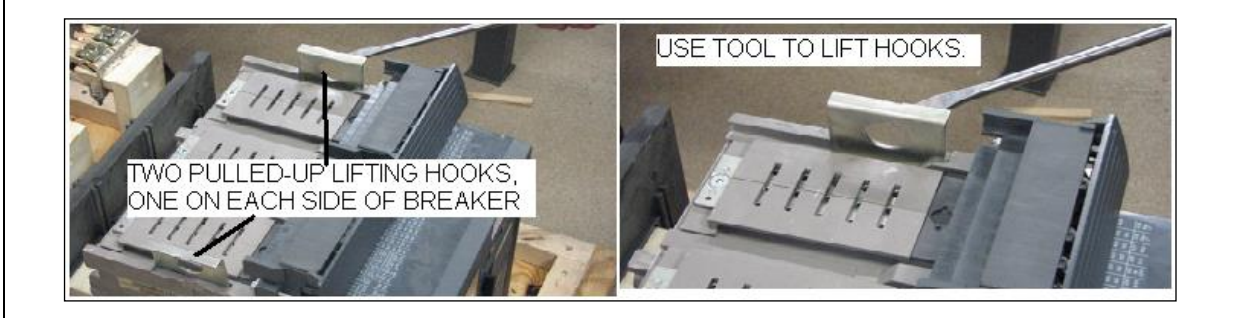
Figure 28. AKD-5—Breaker Lifting Holes
