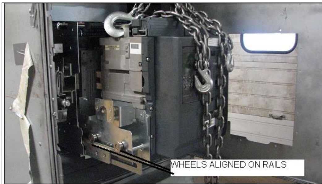
Figure 35. Breaker Positioned on Rails
