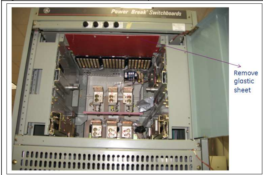
Figure 11. Remove Glastic Sheet – AKR-30S only
