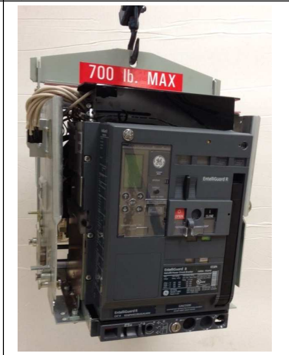
Figure 14. AKD-8—Using GE Lifting bar and hoist
