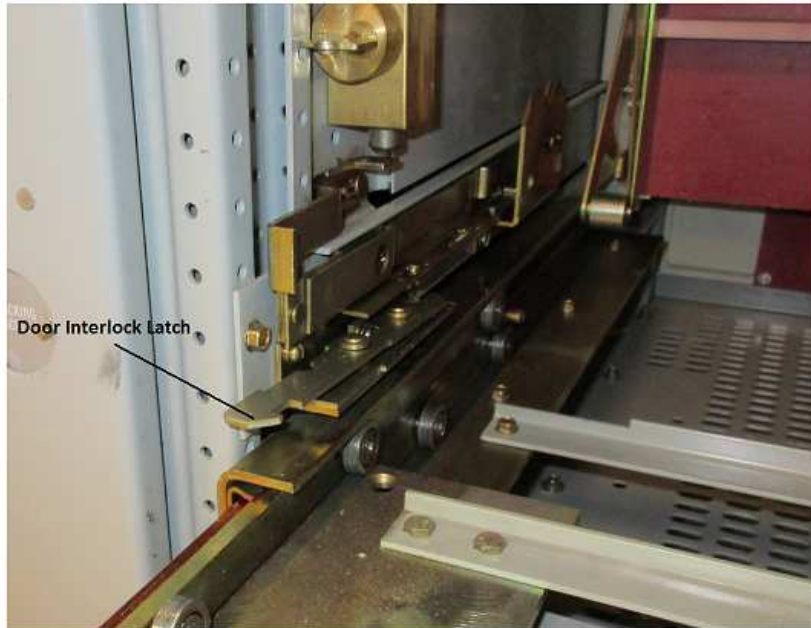
Figure 46. AKD-8 (AKR75/100/125)—Door Interlocking Components
