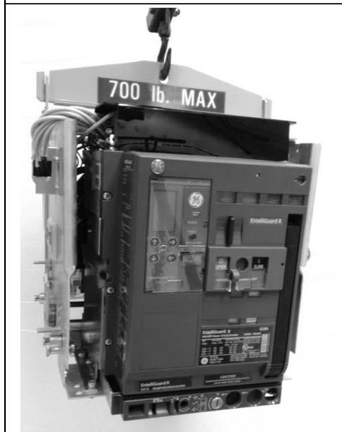
6. Make sure that the lifting bar is secured and locked in place on the breaker. Check that the breaker is free from obstruction inside the compartment.
