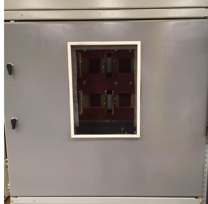
Figure 17B. New Door Assembled on AKD-10— 38"-Door, 5000A
