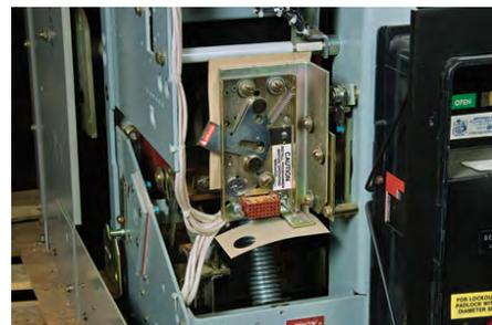
Align the connectors and rejection pin and connect the EntelliGuard TU to the circuit breaker, as shown in Figure 16-3.
