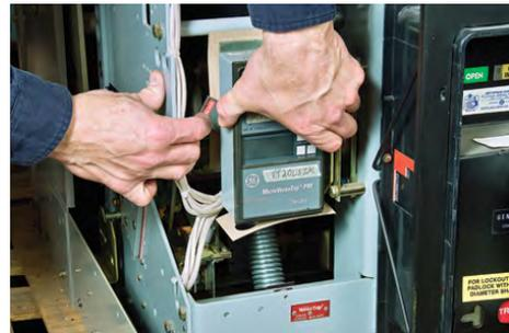
If the breaker is equipped with a MicroVersaTrip RMS 9 trip unit, the 36-pin trip unit connector must be removed and remounted on the adapter bracket provided. Slide the connector out of the mounting plate and install it on the adapter bracket, as shown in Figure 16-2.
