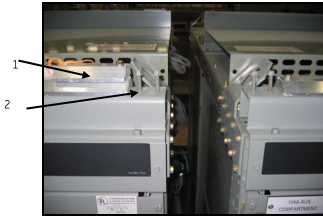
Fig. 4-26. Switchgear shipping split front splice plate
