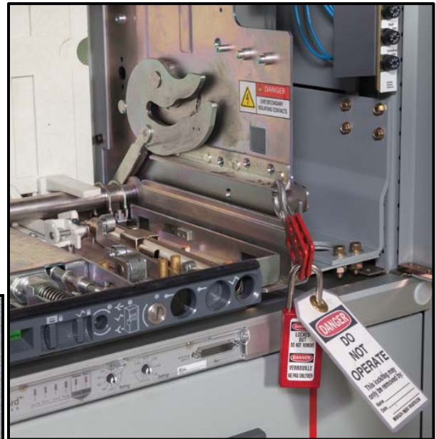
Fig. 7-7. Compartment padlock device
