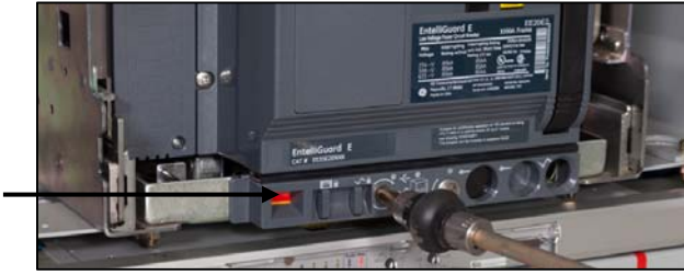
Fig. 5-4. Rotate the racking handle while looking at the indicator barrel
