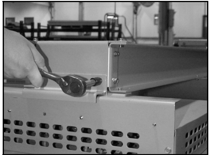
Fig. 4-24. Replacing the runner guide after completion of hoist installation
