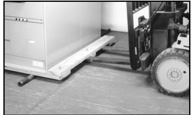
Fig. 2-5. Placement of rollers under shipping skid
