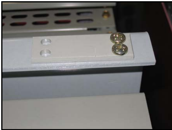
Fig. 4-27. Switchgear shipping split rear splice plate
