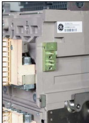
Fig. A1 A breaker pin Assembly
