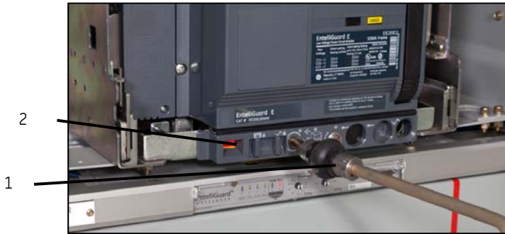
1. Racking handle 2. Breaker position indicator
