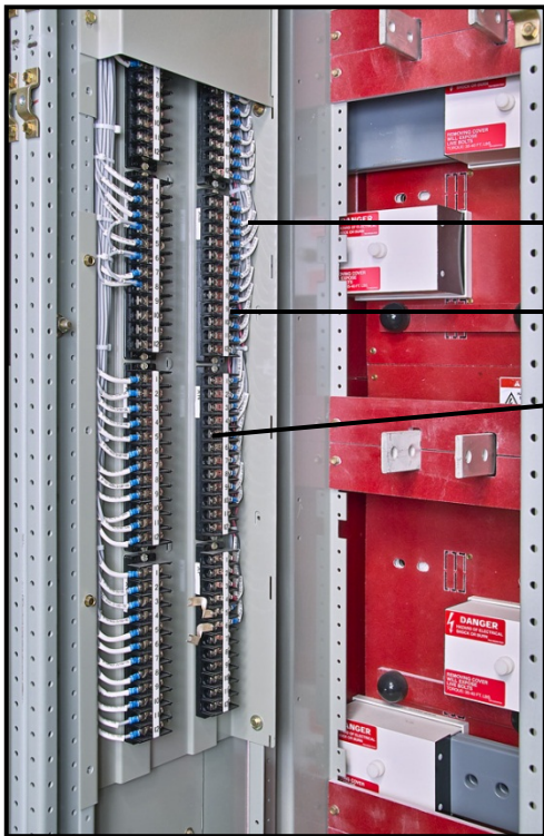
1. Internal equipment control wiring 2. Terminal boards 3. Space for purchaser's field control wiring Fig. 3-20. Control wiring termination trough
