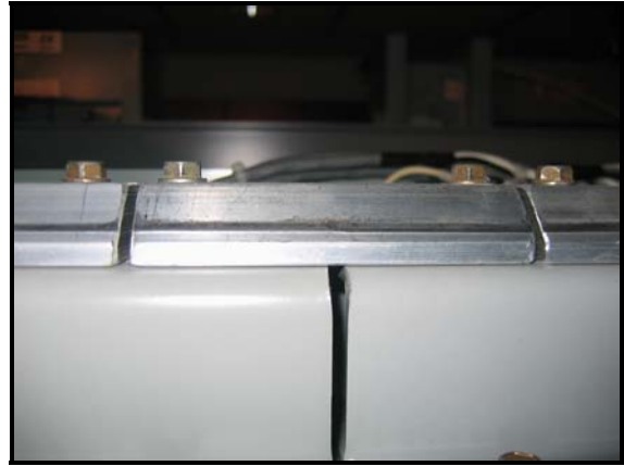
Fig. 4-28. Switchgear shipping split front hoist rail splice plate
