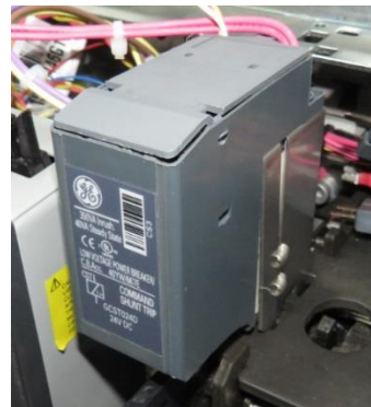
Figure 4. Shunt Trip assembly
