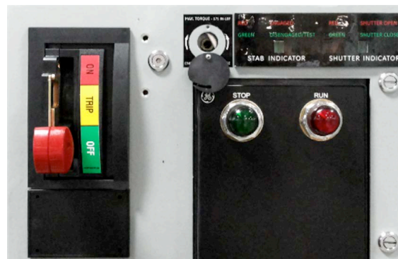
Figure 2c. Lead screw cover after removing from door
