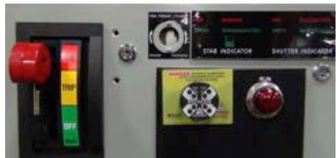
Figure 2b. Lead screw not accessible in disconnect "ON" condition
