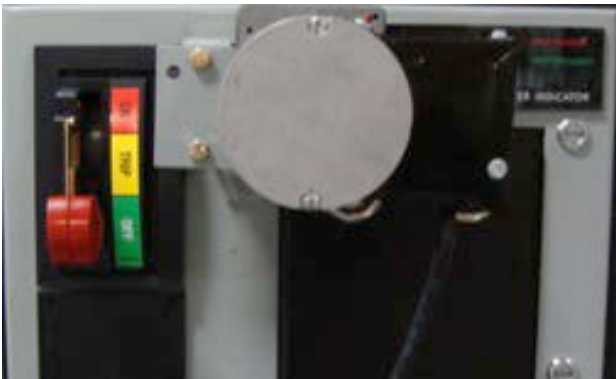
Figure 4b. Assembled condition of motor on door.
