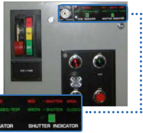
Figure 5. Mechanical Indicators showing DISENGAGED position
