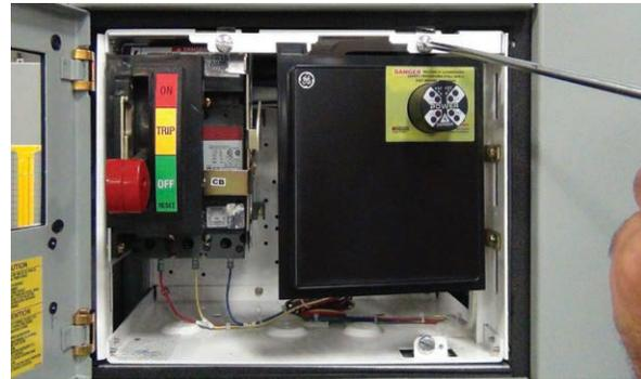
Figure 3. Unlatching the unit
