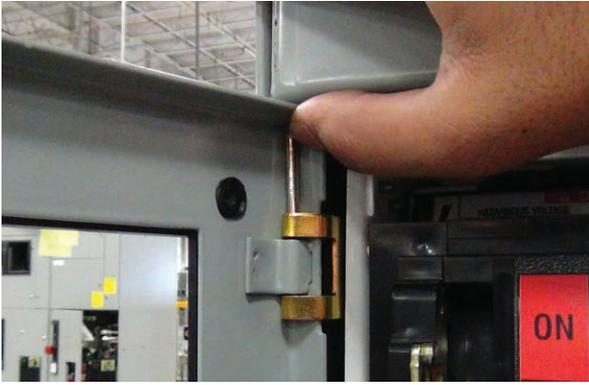
**Figure 5.** Removing the door from the section
