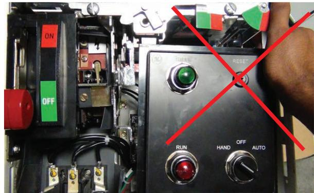
Figure 11. Avoid placing your hand on the shutter indicator while inserting the AFM unit
