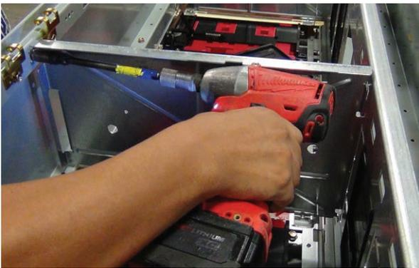
**Figure 6.** Removing shelf from the unit
