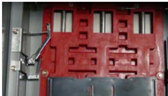
**Figure 9.** Assembling AFM shutter mechanism
