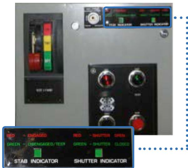
Figure 4. Mechanical indicators showing DISENGAGED position
