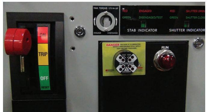
Figure 5b. Lead screw not accessible in disconnect “ON” condition
