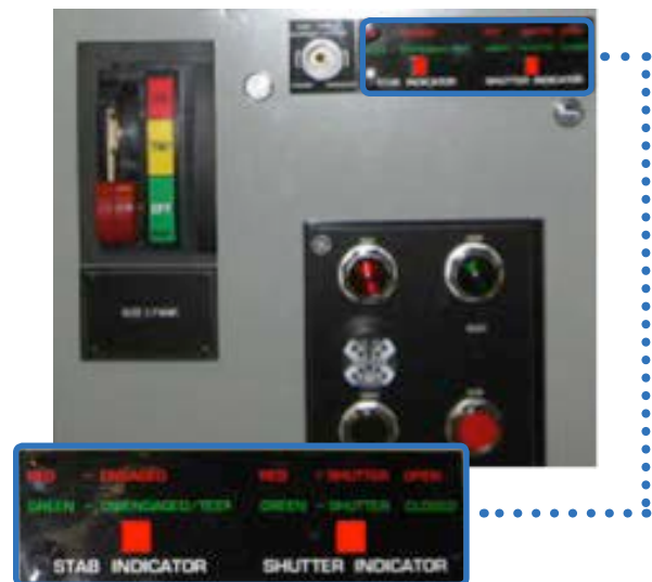
Figure 3. Mechanical indicators showing ENGAGED position
