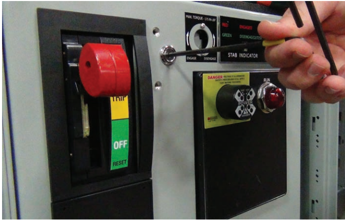
Figure 7. Defeater operation
