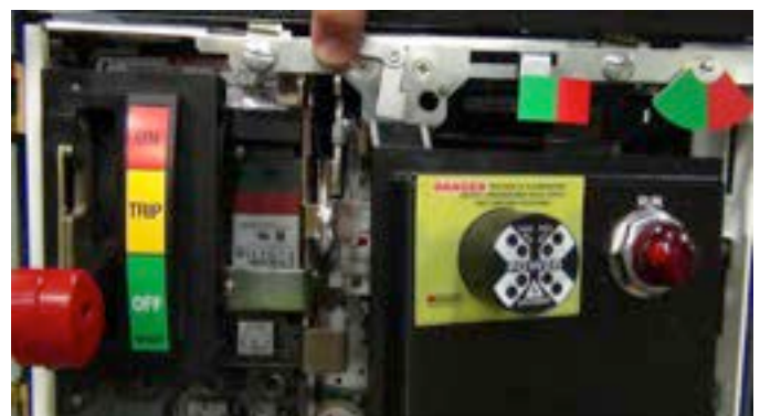
Figure 6. Padlockable lead screw cover
