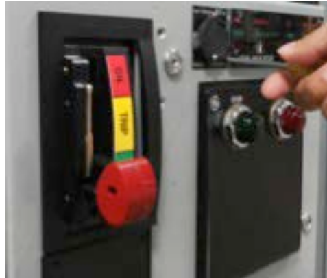
Figure 2. Removing racking screw cover from door
