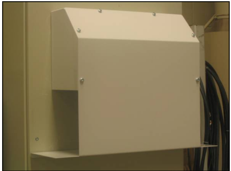
Figure 19. Upper deflector assembly installed
