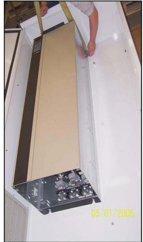
Figure 9. Drive installed in enclosure
