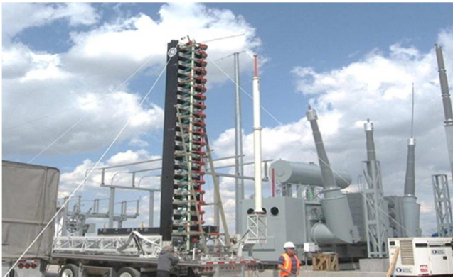
Impulse test of 235MVA/525kV transformer
