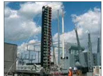
Onsite impulse testing equipment
