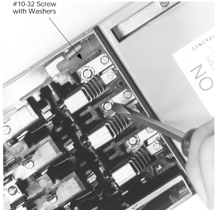
Figure 6. Making the electrical connections.
