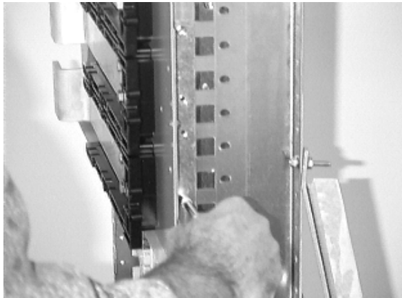
Figure 3. Mounting the switch in position on the interior.
