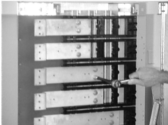
Figure 4. Securing the module straps.
