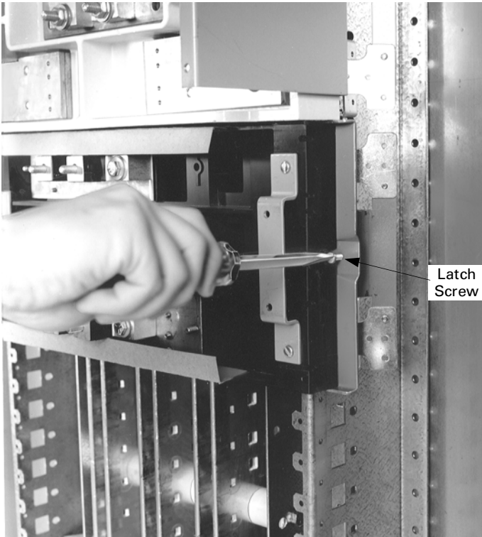
Figure 3. Installing the circuit breaker module.
