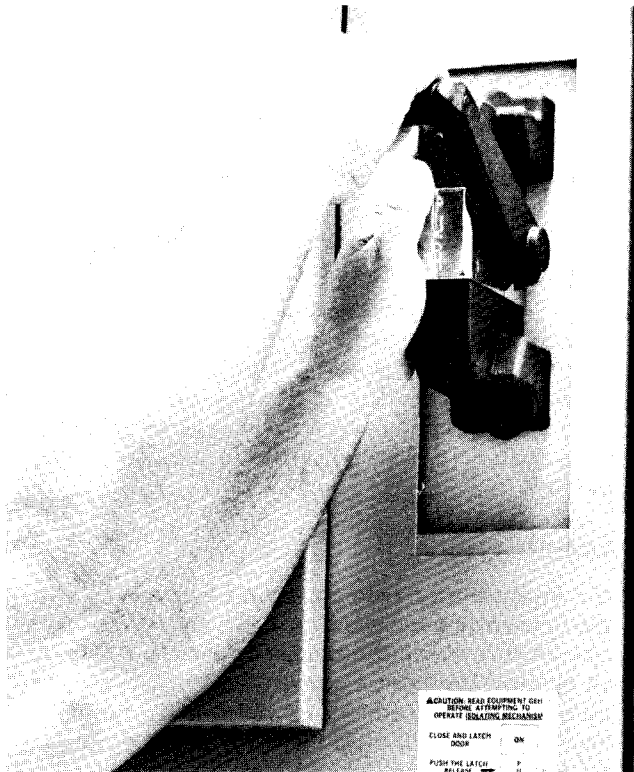
Figure 17. Operate handle by depressing handle latch release with one hand and moving the handle with the other hand.
