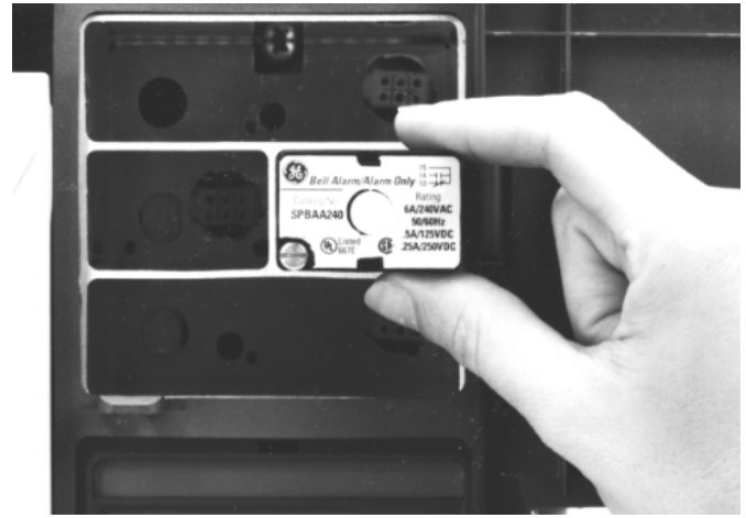
Figure 4. Inserting the Bell Alarm–Alarm Only into the accessory compartment.
