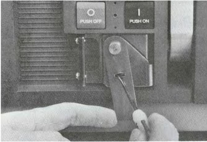
Figure 4. Releasing the locking lever from the interlock spring with the breaker on.
