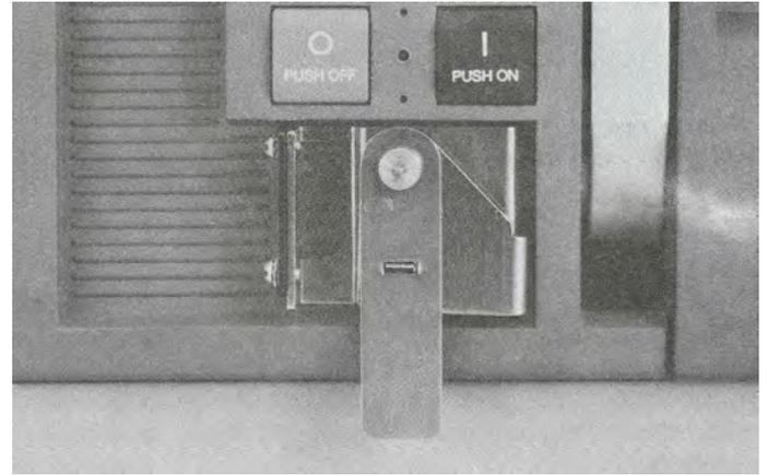
Figure 2. Door Interlock in place to prevent opening the enclosure door.
