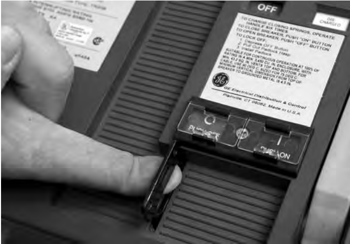
Integral padlock device
