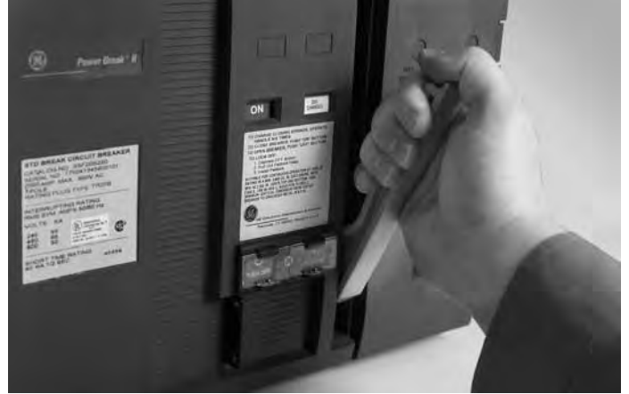
Operation of circuit breaker pump handle
