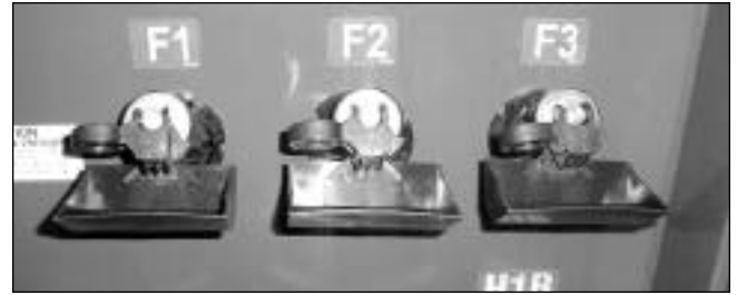
Bayonet with fuse mounted drip shields
